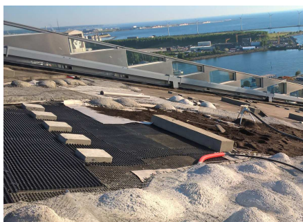
Protectodrain® and Elastodrain® mats ensure the safe drainage of exceeding water on the entire surface.
