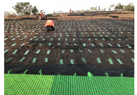
The substrate underneath the plastic mats lies embedded between two layers of geogrids.
